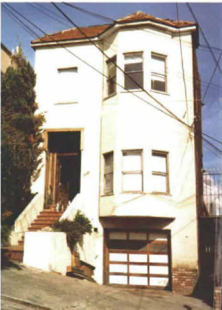
Tiled and defiled. By the 1950s, many San Franciscans had stripped their houses and stuccoed them. This Italianate Victorian had been further disfigured with a barrel-tile roof.
