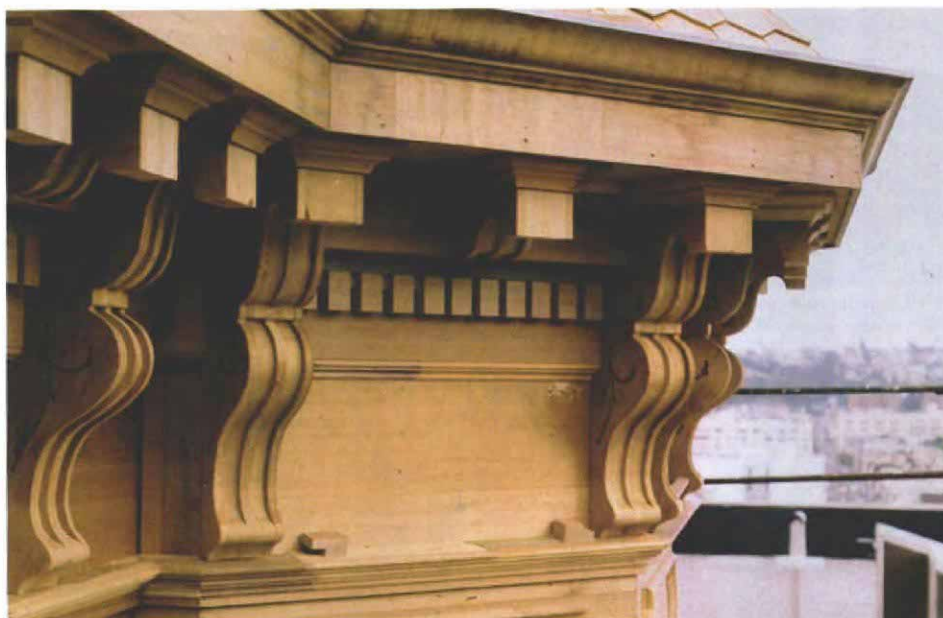
Cabinet-grade trim at 30 ft. Curvy brackets and modillions (smaller brackets), which are laminated from alternating layers of 1x and 2x redwood, detail the cornice's soffit and frieze. The dentils provide a secondary level of texture. On top of the architrave, two dentils await installation.
