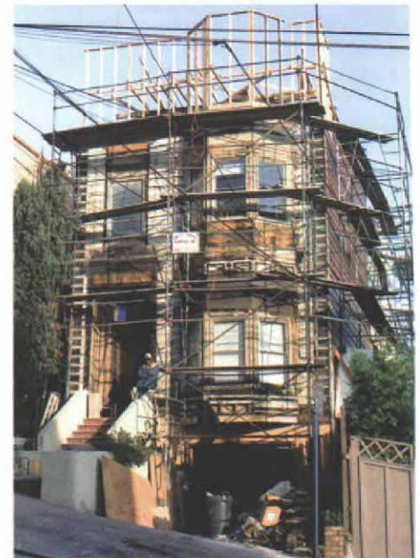
Putting it back. Guided by an old photo of the house, the author extended the parapet and the bay window to their original heights, then began work on the restored cornice (top).
